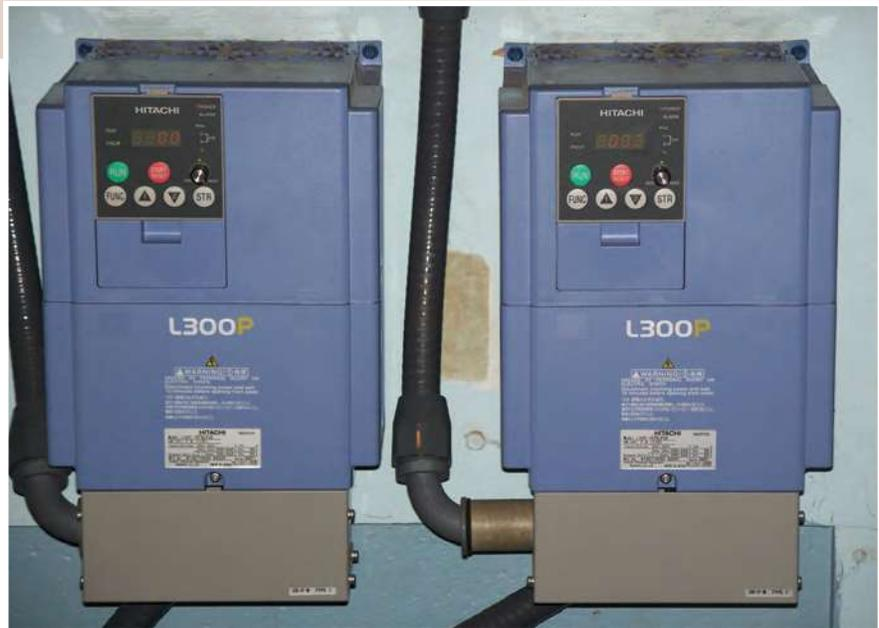
Cherokee RWD 1 installed two VFDs on one of its pump stations a year ago. Costing about \$7,000, the units have eliminated the need for the district to maintain a deteriorated hydro-pneumatic system. The new controls also provide early warning notification of pending problems in the plant.
