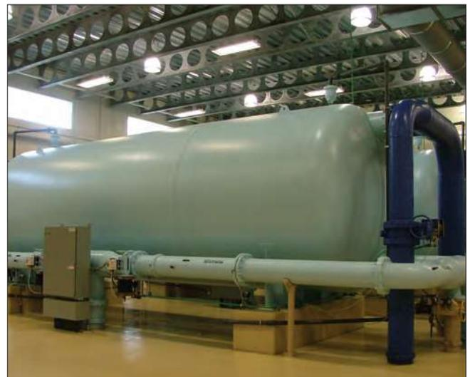
Pretreatment units shown above consist of three pressure filters. Anthracite and greensand media are used to remove iron and manganese, protecting the RO membranes.
