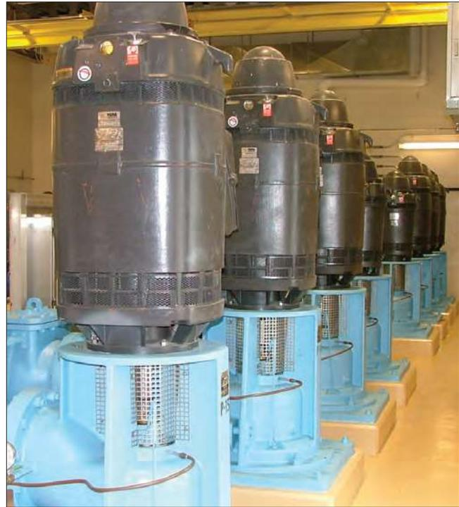
Six of the eight pumps shown here pump treated water to the distribution system. The two pumps in the center of the row are pressure filter backwash pumps.
