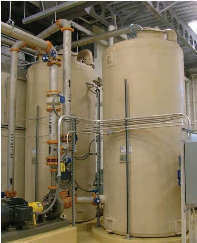
This tank and pump arrangement is the clean-in-place system which uses RO treated water for cleaning the membranes.
