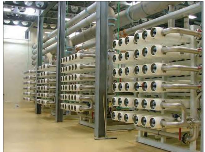
The Hydranautics RO membrane system consists of four skids. Each skid contains 36 tubes with 252 individual membranes. The four skids therefore, have a total of 1,008 eight-inch diameter membranes. The membranes are two stage units.
