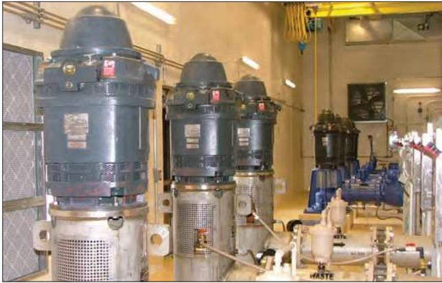
This photo shows two sets of pumps; the nearest pumps with tan piping transfer concentrated reject water to disposal wells. The pumps in the background are the four raw water pumps on variable frequency drives (VFDs).
