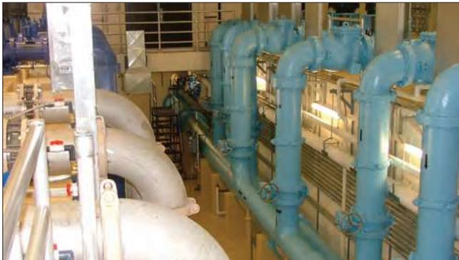
This is a shot of the pump and piping gallery with waste and raw pumps on the left and finished water and pressure filter backwash pumps on the right.
