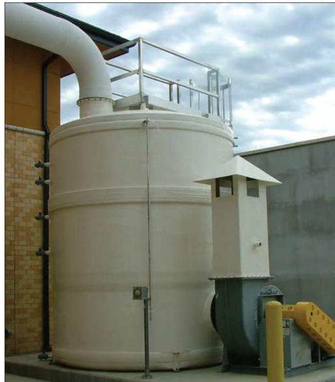
This photo shows the scrubber treatment equipment used to handle the accidental release of chlorine gas. This equipment is usually designed to neutralize and absorb the entire contents of a one-ton cylinder. Please check out the article "Containment systems help ensure chlorine capture" by Gary Armentrout in the July 2004 issue of *The Kansas Lifeline* magazine for more information on this subject.
