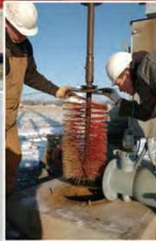
In a well remediation, Alexander Pump's unique truck mounted hydraulic walking beam (above) cycles the surge tank, double surge block and brush (left) up and down through the well. The action forces 'Redi Clean' chemicals into the gravel pack to dissolve iron bacteria, placing it into suspension for removal.
