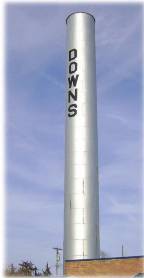
The standpipe serving the city of Downs is one of the oldest, if not the oldest, standpipes in Kansas. Note the tank is riveted steel plates.
