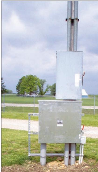
This photo shows the manual switchgear to change from purchased power to emergency power.
