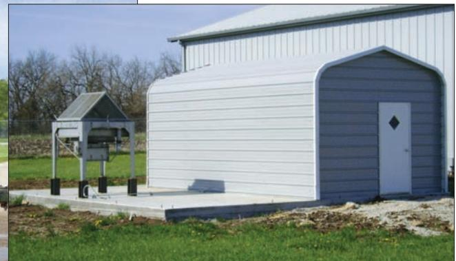
This small building houses the plant generator. Note motor cooling radiator to left of building.
