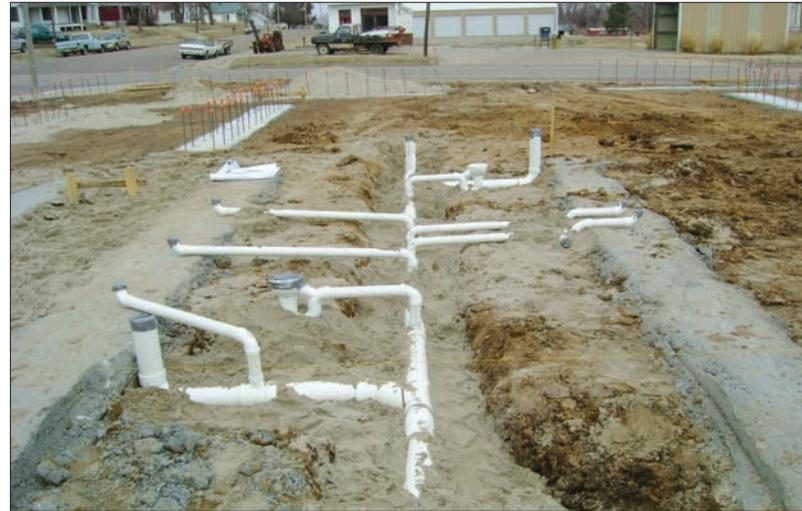
Proper placement of the plumbing is always critical. This photo shows plumbing for the restrooms before being back-filled. One toilet, one sink, one drain – and one shower. Simple and practical – as it should be.
