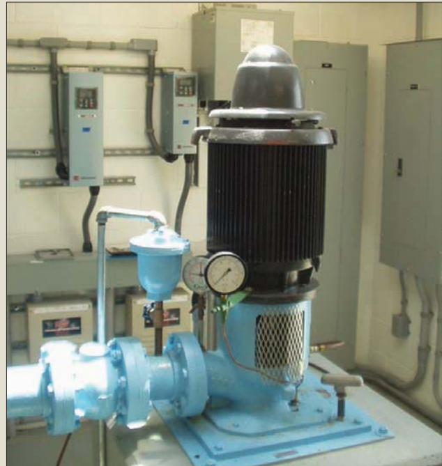
This photo shows a typical vertical turbine pump on a municipal water well in northeast Kansas. The well is adequately sealed; the vent is screened to prevent entrance of contaminants.
