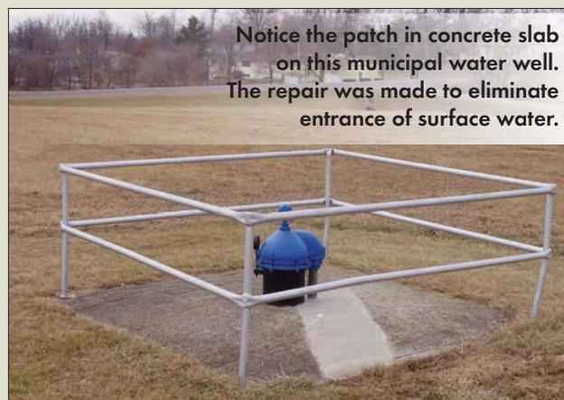
Notice the patch in concrete slab on this municipal water well. The repair was made to eliminate entrance of surface water.
