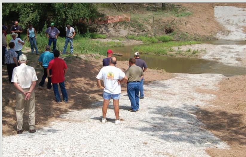
This hardened stream crossing through Big Creek in Russell County was constructed to give livestock access to water and to grass on the other side of the creek, without damaging the streambanks. It is also designed to encourage livestock to leave the stream after drinking.
