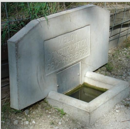
These sturdy concrete livestock waterers have a small reservoir at ground level. The reservoir extends behind the concrete back to help keep the water from freezing in the winter months. Removing two screws easily accesses a float valve and a shut-off valve behind the metal plate.
