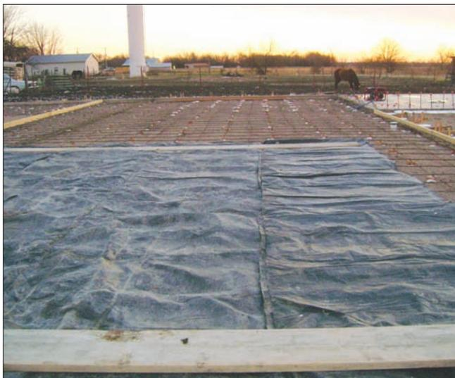
**Temperatures were expected to drop to the lower 20's on December 10, 2008. The sub-grade on the Fire Station in Dennis, KS was covered to allow a pour the next morning. Concrete can be poured during colder weather conditions but necessary precautions need to be taken.**
