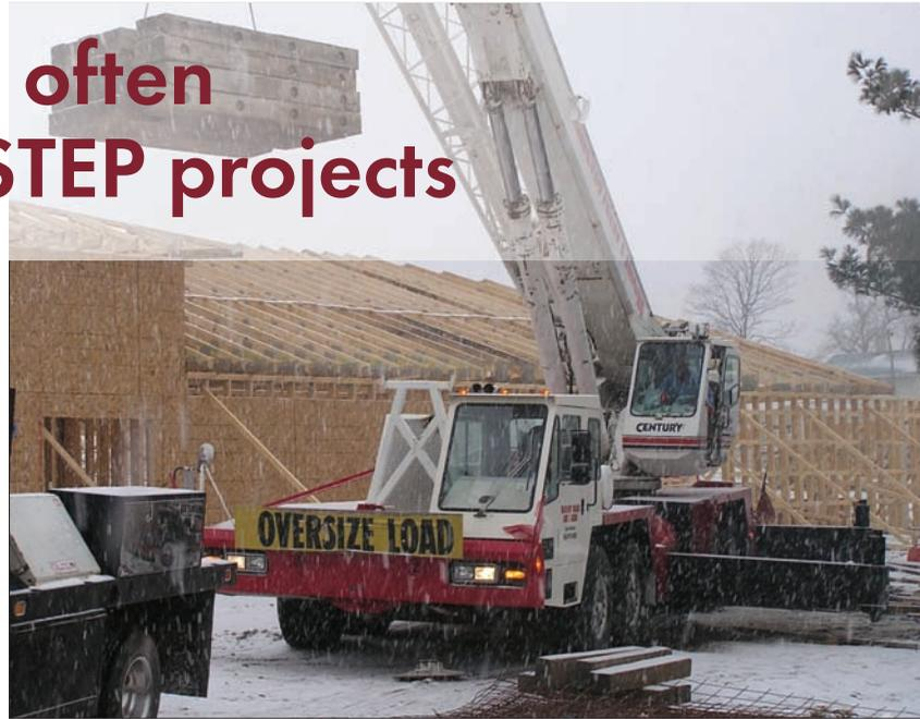
Even snow can slow down progress when setting trusses. The crane operator on the city of Highland’s KAN STEP fire station just finished setting the last truss and is loading the outrigger supports.
