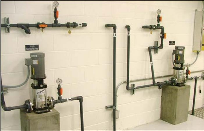
*These booster pumps are for pre- and post-chlorination. Pre-chlorination is used to oxidize the iron and manganese and post-chlorination is used to maintain the desired chlorine residual in the distribution system.*
