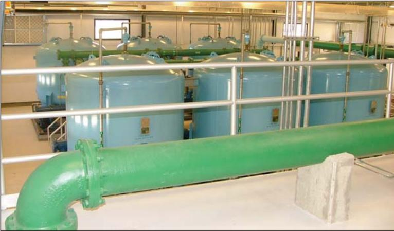
Taken from the mezzanine section of the water plant, this is an overhead view of the Layne Ox pressure filter layout.
