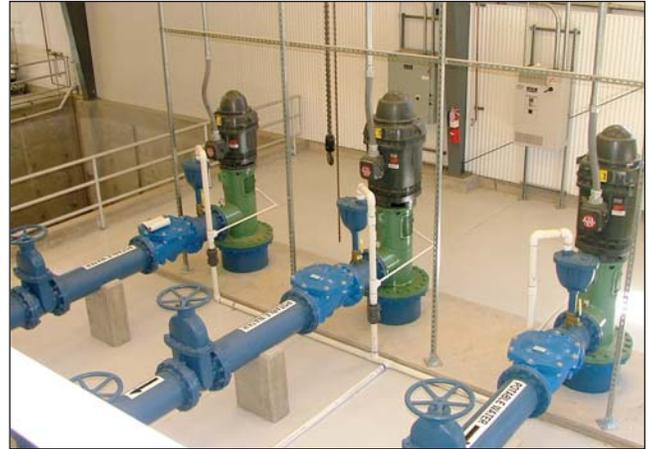
This is a view of the pumping system in the plant. The two pumps on the right are high service pumps that deliver water from the clearwell to the distribution system. The pump on the left is the backwash pump.
