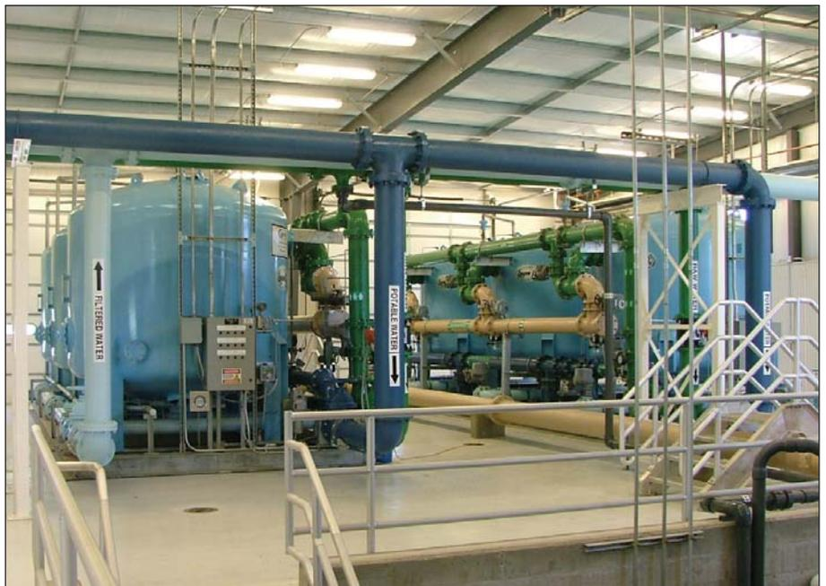
*This end view of the pressure filter vessels shows the piping system. The green piping allows raw well water to enter the plant; the light blue piping allows filtered water to leave the filters; the dark blue piping allows treated water to be used to backwash the filters.*
