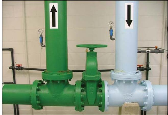
*This connection allows raw water to bypass the plant. The green pipe on the left is the raw well water line to the filters. The light blue line is the filtered water line (treated water) from filters. The valve between the two lines is normally closed but can be opened if there is ever a need to bypass the plant.*
