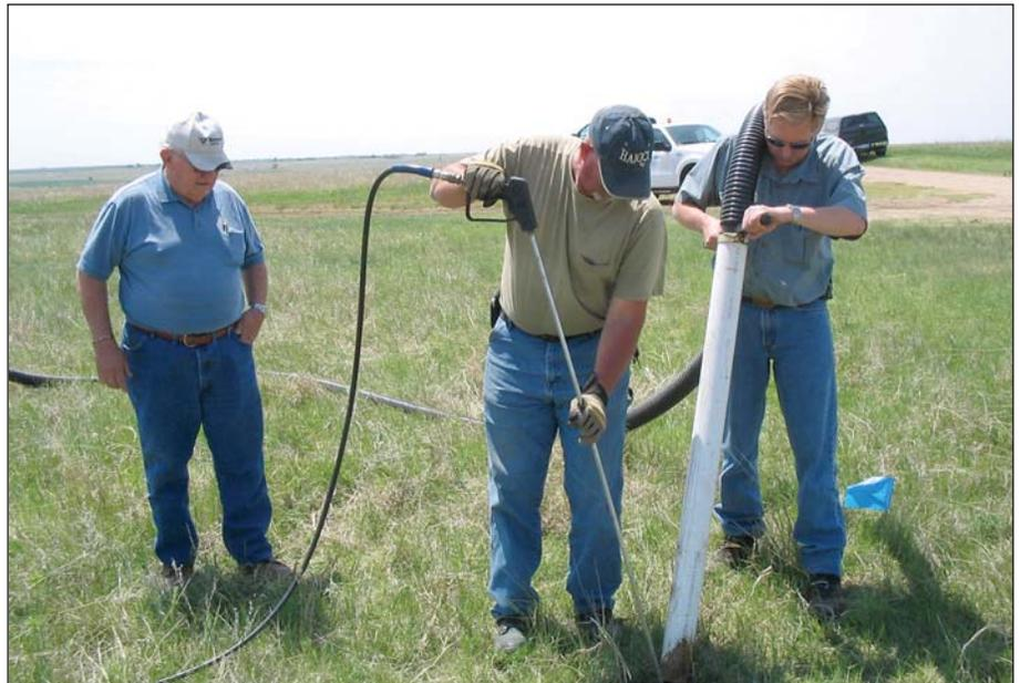
*In the picture above a Vermeer potholer factory representative (left) observes Russell RWD 3 Manager Ron Nuss as he directs the power gun while KRWA Tech Doug Guenther runs the vacuum boom. They are working to expose and locate a water main to be crossed by a fiber optic cable crew working in the RWD territory.*
