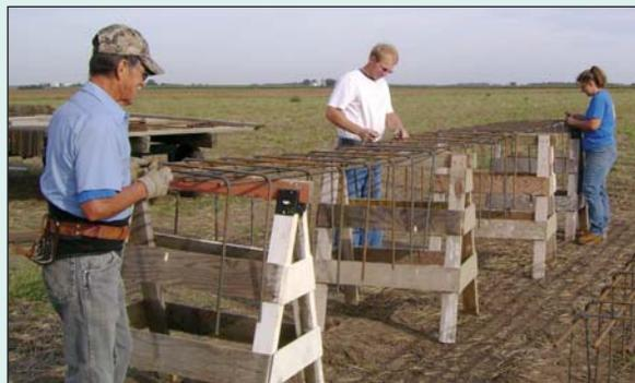
The rebar that goes into a footing is more easily assembled above ground. Here, a section of the 'cage' for the new KAN STEP Fire Station at St. Joe in Reno County is being tied by volunteer Jim Weinman, KRWA Tech Mike Fisher and volunteer Kendra Ernst; another section has just been completed.
