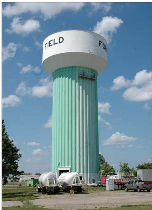
recirculation pump with the method of adding combined chlorine at the top of the water storage also has merit. In this case, the rate of circulation in gallons per minute is important. In either case, reducing the amount of water stored (say, 0.35 MG) will make each method more effective. The operations of the tank (water levels, rechlorination levels, recirculation rates) are all important to the success of maintaining chlorine residuals in such a large tank."
