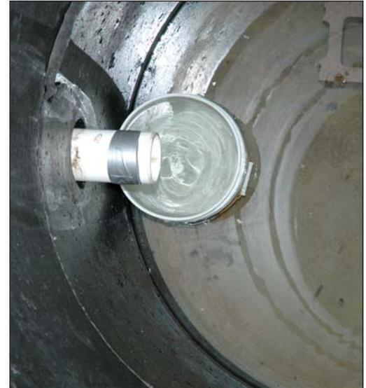
Seen above is the manhole where water that seeps through the first liner collects. Current seepage rate is about two gallons per month, well within KDHE specifications according to Don Hellar. Don stated that a pump will be obtained to return the seepage water to the lagoon.
