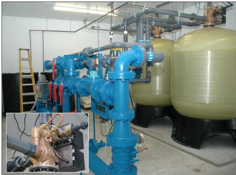
Pictured above are the two ion exchange tanks with related piping system. The tanks contain nitrate selective resin provided by Krudico, Inc., and the piping system within the tanks was supplied by Pentair Water Treatment. In the background are two brine tanks and one of the city's well pumps. **Inset:** Pictured is an enlarged view of one of the automatic control valves located on top of the ion exchange tanks. Automatic operation is based on flow through the plant.
