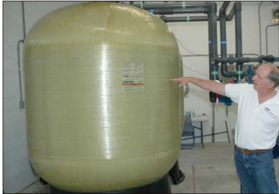
**Far left:** Don Hellar, Project Engineer, removes the cover from one of the brine tanks to display the salt brine solution used to regenerate the resin in the ion exchange tanks. **Left:** Don Hellar points out the approximate level of the resin in the ion exchange tank.
