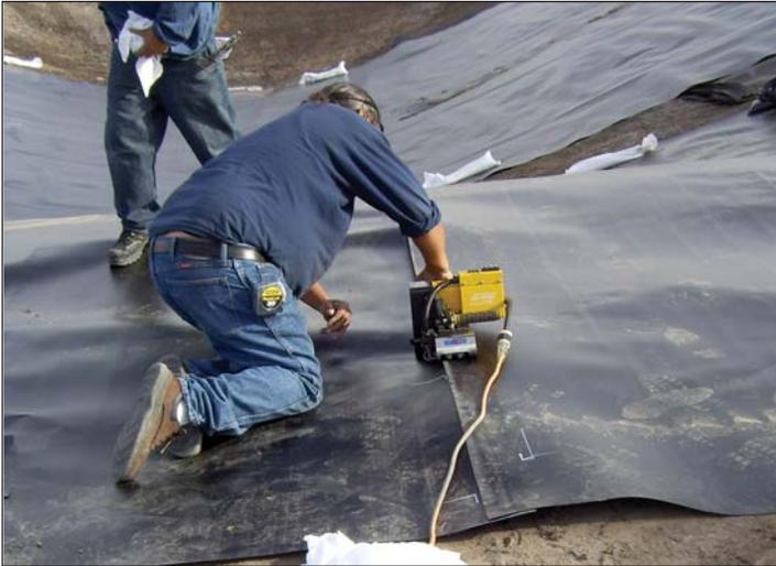
The photo above shows workers on the lagoon project sealing the HDPE liner joints.
