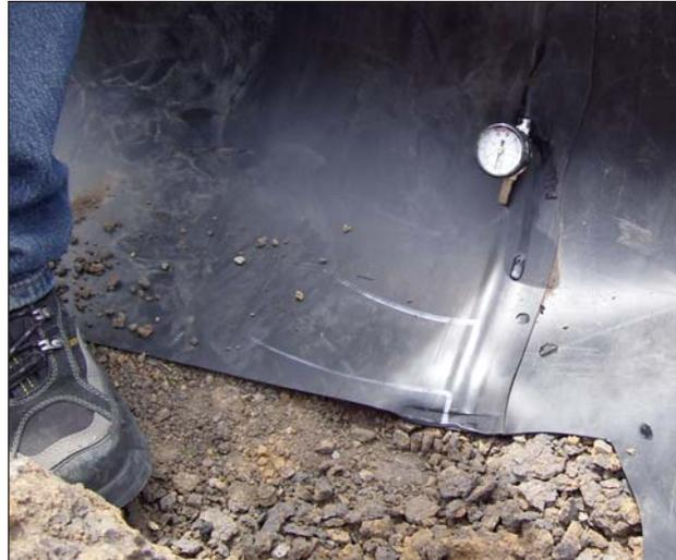
Seen above is the pressure gauge that was used to confirm that the HDPE liner joints on the lagoon liner were adequately sealed.
