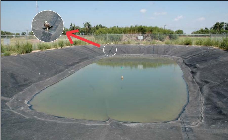
Shown here is the double lined lagoon used to contain the concentrated nitrate and brine waste water. Note the attraction to wildlife, the hawk, located in the small circle and seen close-up in the inset and the rather significant security fence. Don Hellar noted that deer are the most serious hazard to the synthetic liners, as their hooves will damage the liner causing it to leak.
