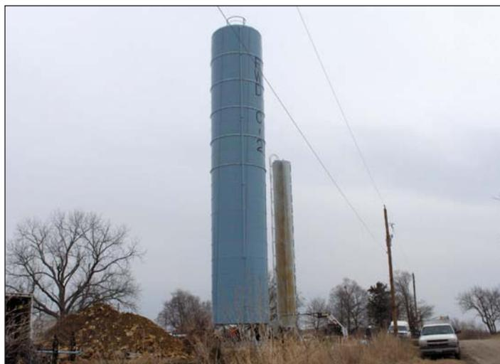
**Left:** The new Bourbon Cons. RWD 2 storage tank is seen reaching skyward as the construction crew assembles another ring.
