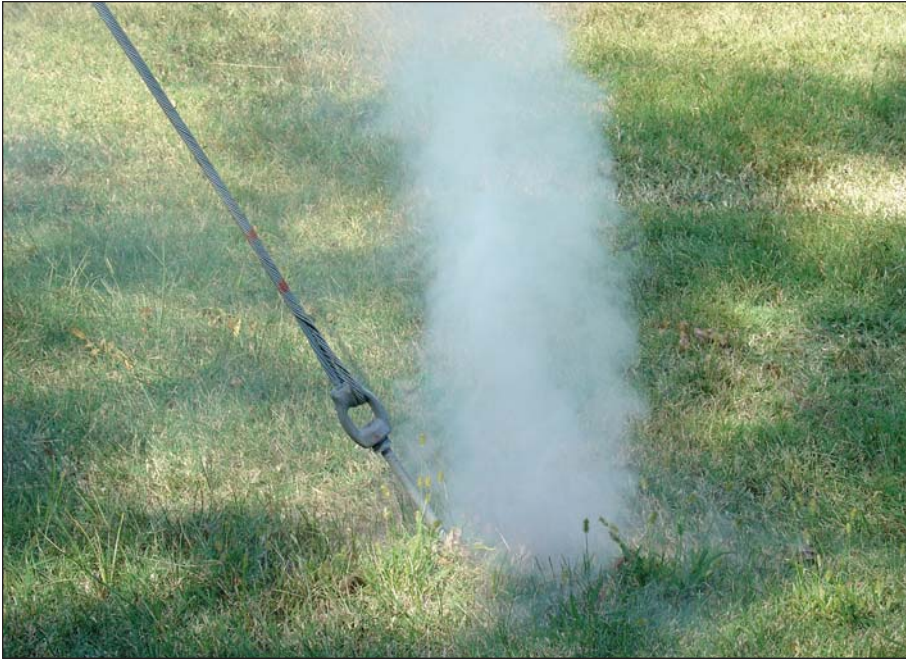
Smoke escapes from a service line where the electric utility placed their anchor.
