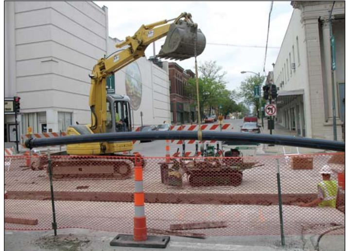
Water Department Manager Don Murphy explains. "Our crews also favor the new pipe over ductile iron because of the ease of installing the pipe and the fact that even with the larger size pipe, there are no gaskets to worry about leaking. The larger size pipe is fused together at the joints. This fusion of pipe eliminates the need for a gasket and the possible leak point in the future."
