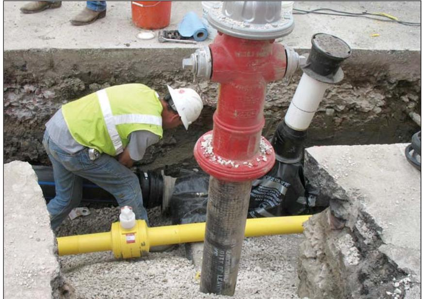
**Left:** The 8-inch HDPE pipe is seen placed in the trench threaded under utility lines that pass above. A 3-foot clearance must be maintained between all of these utility intersections. The yellow line lying on the left above the trench is a gas line being pressure tested before placement below. The 8-inch HDPE will be shoved to the left trench wall and the yellow gas line will then be placed to the right or opposite trench wall.
