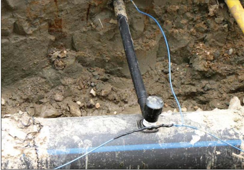
A service connection is shown in the photo above with blue tracer wires following each of the lines. The service connection tap has been electro fused to the 8-inch HDPE for a solid, leak proof connection.
