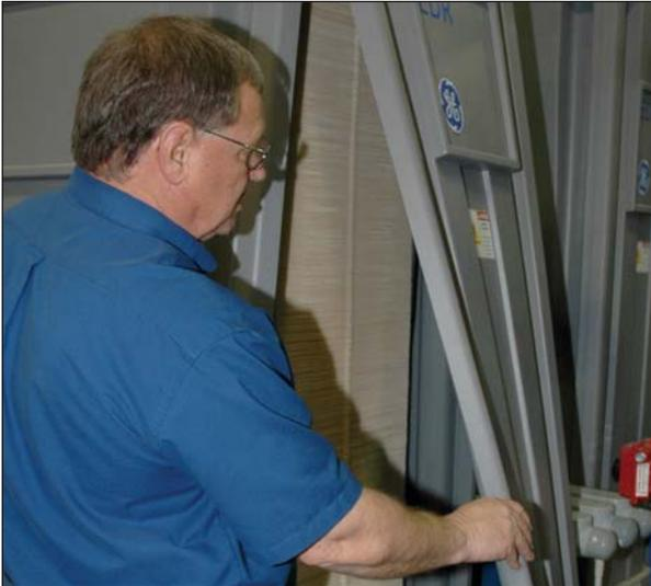
EDR membrane units. GE Water & Process Technologies supplied the units at Russell. The EDR plant layout has eight trains in two individual units (four trains per unit). There are three stack pairs per train. The stacks each contain about 600
