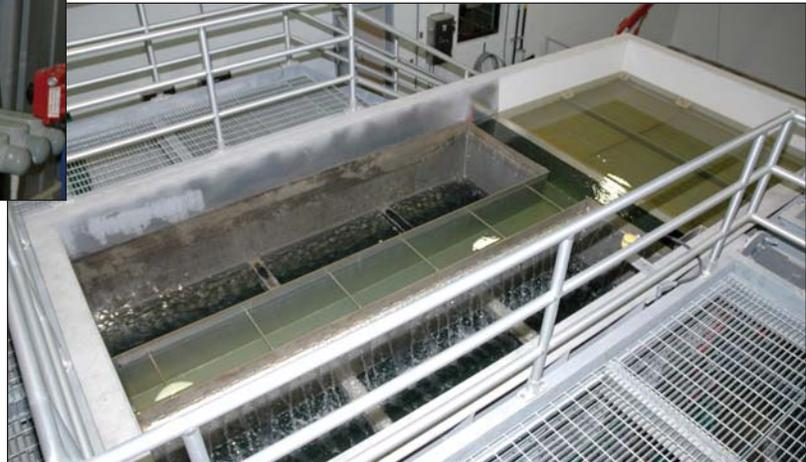
**Above:** The trains are composed of stacks of membranes. Arlyn Unrein, Public Works Director, opens the end of an EDR unit showing the stack of membranes that removes total hardness.
