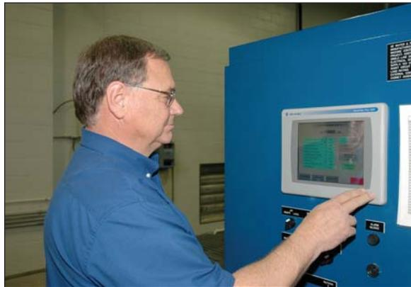
*Left: Russell Public Works Director Arlyn Unrein explains that operators can control finished water quality by adjusting the amount of electricity being applied to the EDR units.*
