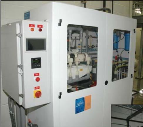
**Left:** The chlorine dioxide generator is shown in the main plant room. Chlorine dioxide is being used to oxidize iron and manganese for removal later.
