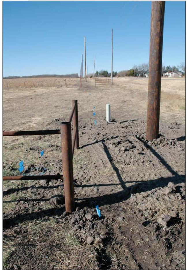
*This busy easement is located south of Wichita and involved a Sedgwick RWD 3 pipeline. The locate flags represented one of many separate locates provided by RWD staff during a two-lane to four-lane road project involving multiple utilities in the easement.*
