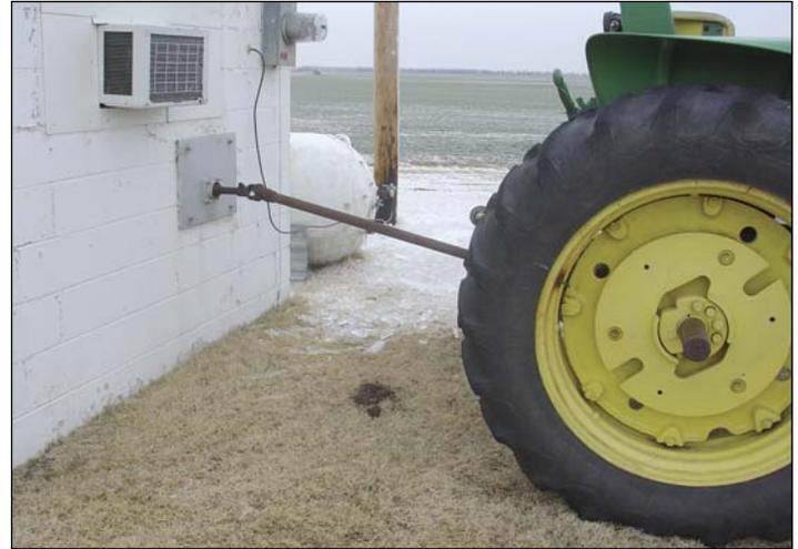
**Above:** A tractor's power take-off or PTO drive is used to run a generator to power one of the Abbeyville, Kan. sewer lift stations.
