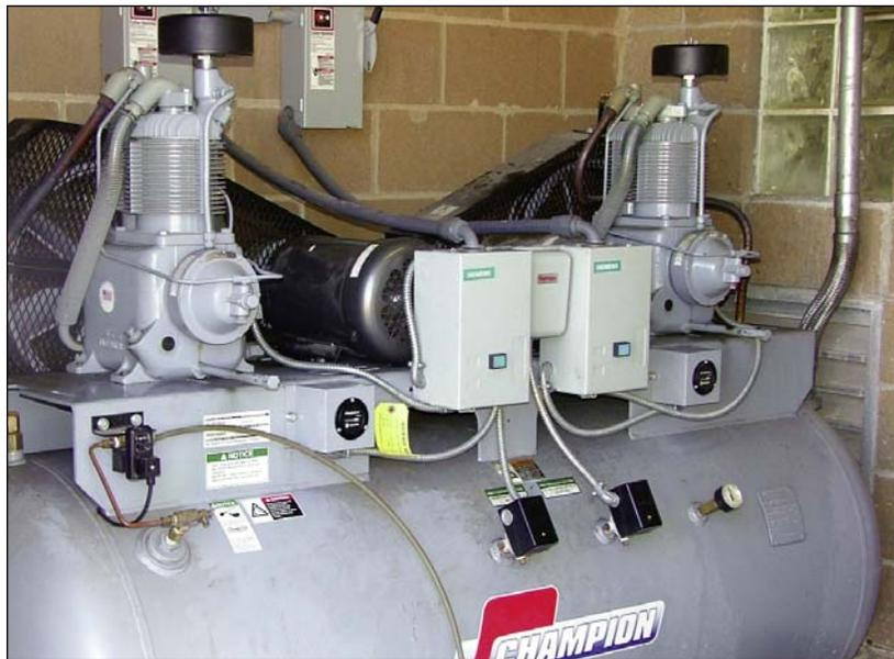
Compressors and pressure tank are used to control pneumatic valves in the plant at Florence
