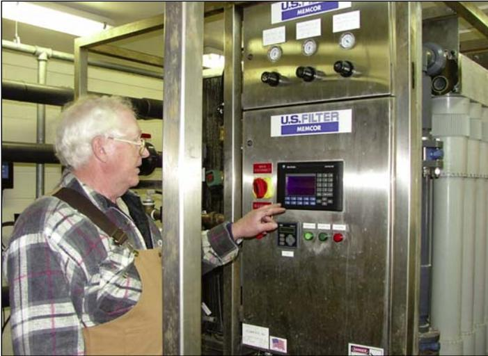
**Left:** Florence Water Plant Operator Larry Scriven uses the computer that controls plant operation. It sits at the end of the Microfiltration skid built by U.S. Filter for the Florence treatment plant.
