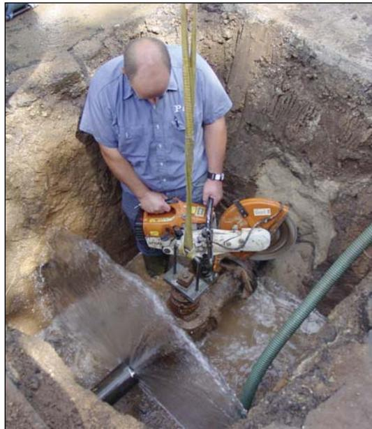
Enterprise City Superintendent Paul Froelich's work to replace a 6-in. valve was part of the Enterprise KAN STEP project. The image shows him making a line cut in the process to remove the old valve. This picture was taken on June 10, 2003.
