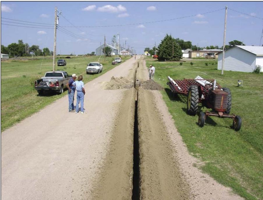
*Local volunteers on the Agra KAN STEP water system project not only proved they can cut a straight trench, the system has not experienced a single leak since installation in 2005. Agra’s project was also an “all new” system, involving pipeline and valves, hydrants and approximately 140 new services.*
