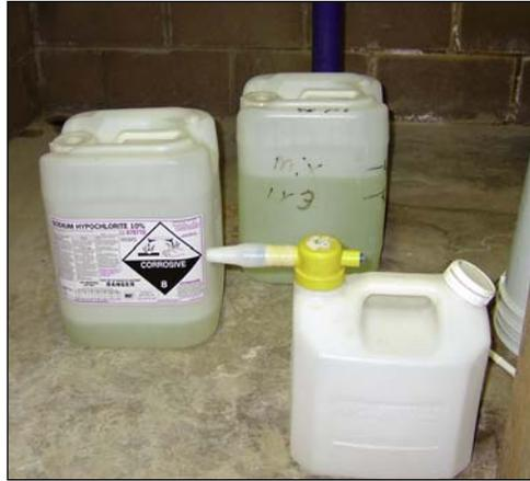
*The sodium hypochlorite solution tank and pump at left and sodium hypochlorite mixing and dilution system above are located in the pump station. Liquid sodium hypochlorite was chosen over gas chlorination because the pumping station was not constructed with a separate room for the safe storage of the chlorine gas cylinders.*
