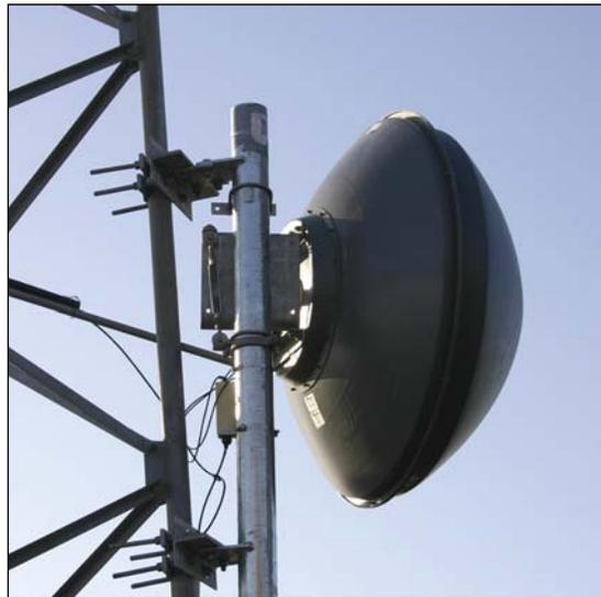
*This is a typical 4-foot in diameter antenna mounted on a structure leg.*
