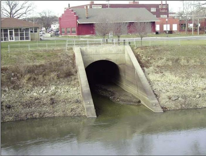
**Above:** The concrete horseshoe CSO discharge location can be seen from the Amelia Earhart bridge. This is a view from the east looking into Atchison. This is actually the outlet for the White Clay Creek but it carries the overflows from 4th, 6th, 7th, 11th and 14th Streets in addition to natural creek water.
