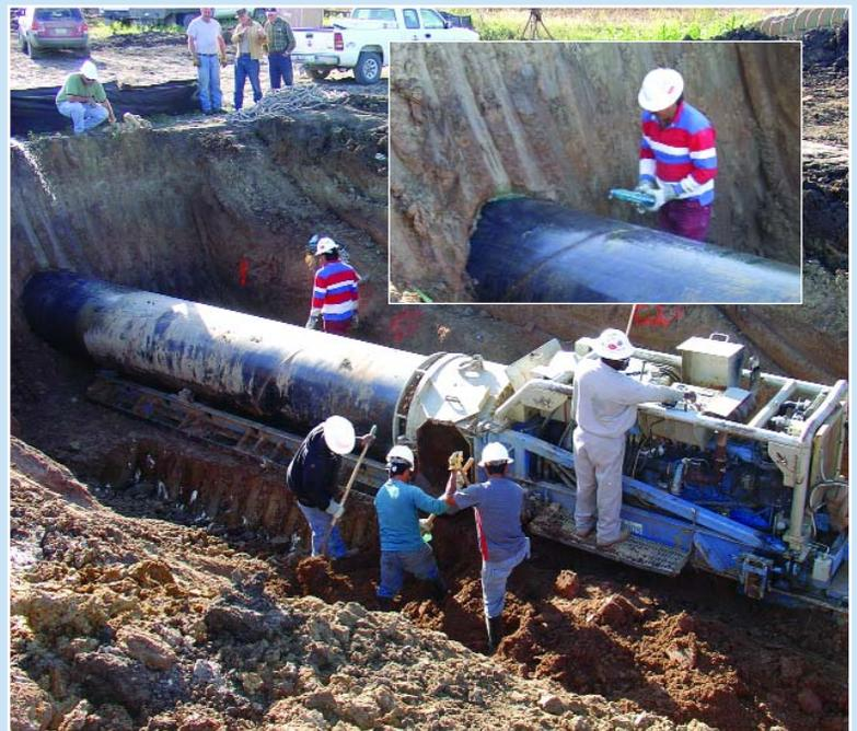
*Above:* Workers bore a township road to install a segment of the REX pipeline. This machine drives an auger inside the casing; workers clear the drilling from the machine. *Inset:* What's the secret? Dawn's liquid soap is applied for lubricant as the bore is made.
