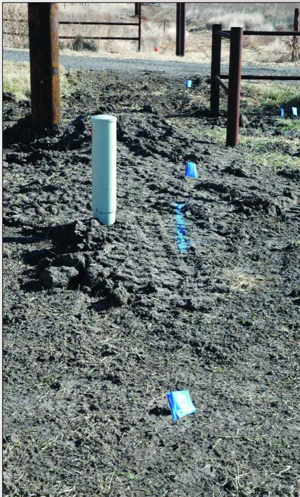
*The photo shows a telecom can in the easement mix. Also located in this stretch of south Wichita easement, besides the rural water line, are power lines, a gas line, both telephone and cable television lines. All these associated utilities jockeying for the same space can cause a real headache.*
