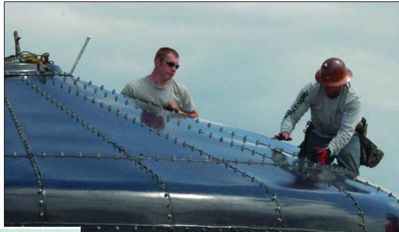
*The storage tank for Phillips County RWD 1 is a 100,000-gallon glass-fused-to-steel Aquastore system. The District chose this style with the expectation that it will give years of maintenance free service. It was erected in just over one week; the cost was \$165,000. The contractor was EAI International.*
