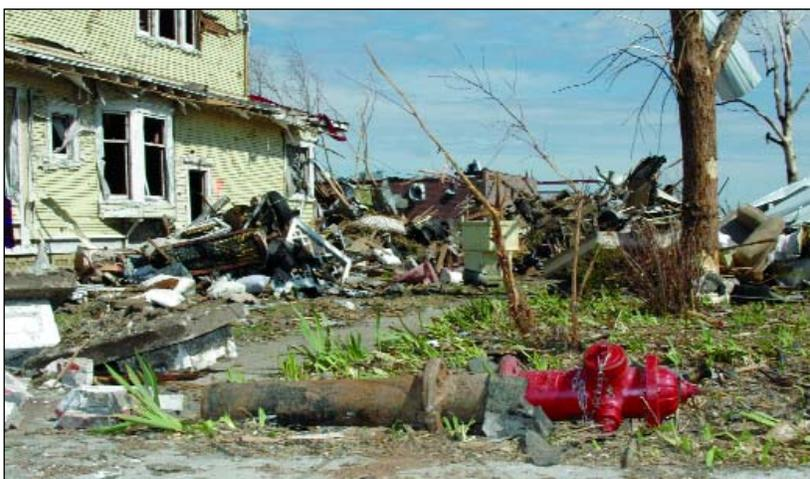
*Left: Better to have this steel stake marker bent than the hydrant to be hit by cleanup crews. KRWA and KMEA members located more than 1000 water meters, hydrants and valves in Greensburg to hopefully prevent further damage to the system.*
