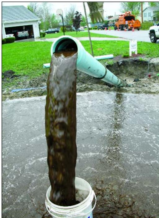
*The concentration of buildup is evident coming from the inside of a ductile iron main. After years of operation and depending on water quality, excessive mineral deposits often build up inside waterlines. Pigging can often remove the deposits, improving water quality and flow characteristics.*
