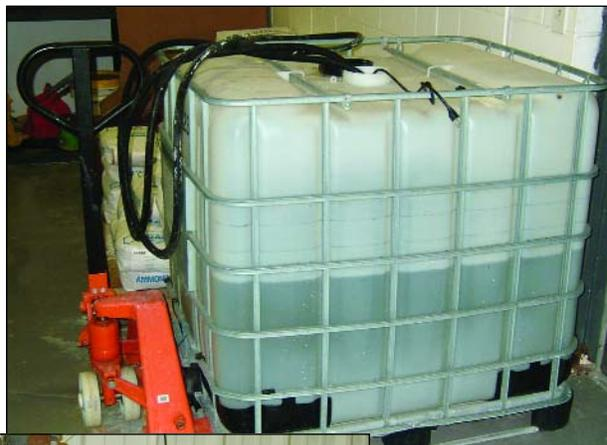
*Left: Granular ammonium sulfate is added to water to make the chemical feed solution. A small solution feed pump is used to add the solution to the water being treated.*
