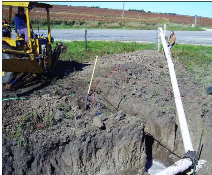
The contractor's tractor anchors the 8-inch line in place with a log chain. The set-up will serve as the pigging project flush point.
