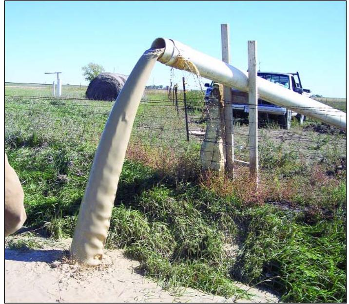
**Above:** The last of the pigs, seen here still in the air, have exited the pipeline. The other two are seen on the ground below the pipe.
