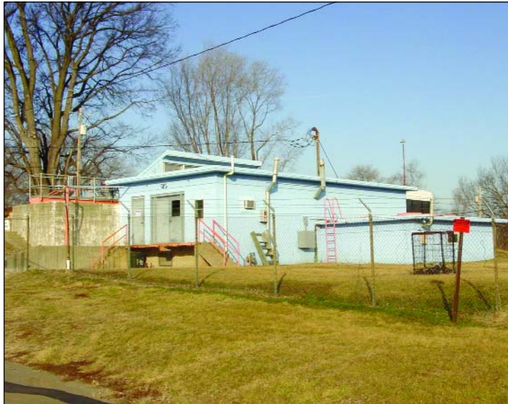
This photo shows the existing water treatment plant in Valley Falls. The city is planning for major improvements to meet SDWA regs and add some capacity.
