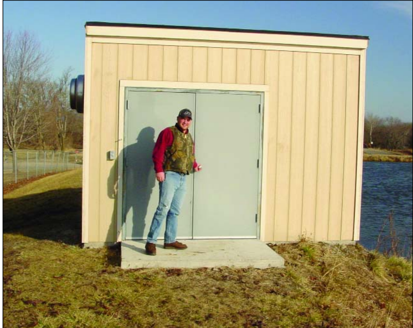
To reduce costs, the city of Valley Falls employees constructed a building at the water impoundment to house the potassium permanganate chemical feed system and the low service pumps. They also intend to construct a building separate from the plant for the activated carbon feed equipment. This will help control the carbon dust problem they are presently experiencing in the plant. Operator Shannon Shields is shown outside the potassium permanganate building.
