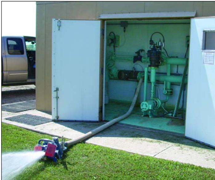
*This booster station is set up to allow the master meter to be tested “in place.” A test port allows for KRWA’s test meter to be placed downstream of the system’s master meter with no need to remove the large meter from its normal position.*
