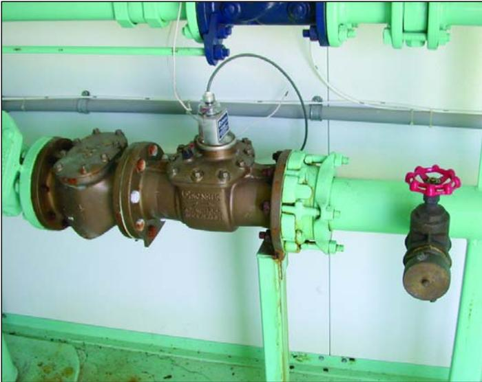
*This installation shows a screen attached directly to a 2-inch meter. Down stream from the meter a 2-inch valve is attached so that the meter can be tested in place.*
