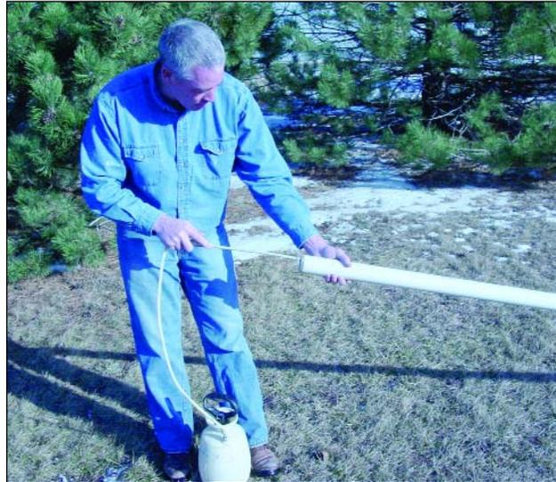
Nemaha RWD 3 manager Paul Strathman demonstrates how he uses a garden sprayer to chlorinate pipe. The HTP solution in the sprayer can be introduced with minimal spillage and mess.
