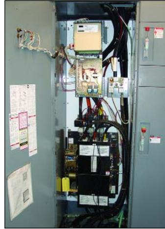
**Above:** This lift station is equipped with a generator connection. If power is lost a portable generator can be used to bring the lift station back into service. The generator can be used at more than one lift station. (Note blue adapter for quick connection.) **Above right:** This disconnect switch will disconnect normal electric power and switch to back up power automatically. It is good to make sure a system is ready to switch if the need arises.
