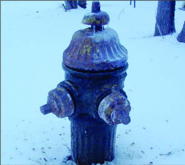
*This hydrant stands as a testament to the importance of a proper hydrant maintenance program. Note the ice on the hydrant and the green color down the barrel. Both are due to water leaking out of the hydrant. This hydrant is located in a residential area across the street from a daycare facility.*
