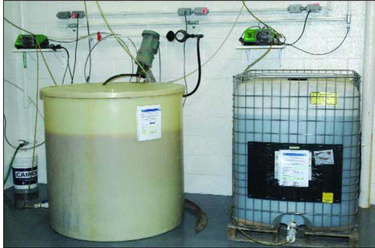
**Left:** New to the plant is the powder activated carbon feeder. The unit's crane can lift the larger half-ton bulk bags of carbon, saving operator time.
