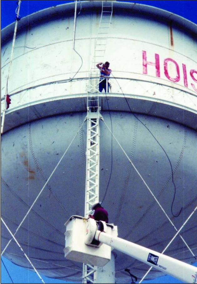
**Left:** A crew from Larned repairs antennae on the elevated water storage tank to restore communications to emergency workers in Hoisington. Note the new "curve" in the ladder behind the worker on the tank catwalk.
