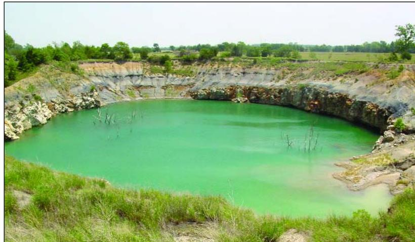
*This image reflects what can happen to undermined areas where inadequate support is left in place. The cities of Treece, Kan. and Picher, Okla. are both in danger of experiencing subsidence such as this in residential areas of the communities.*
