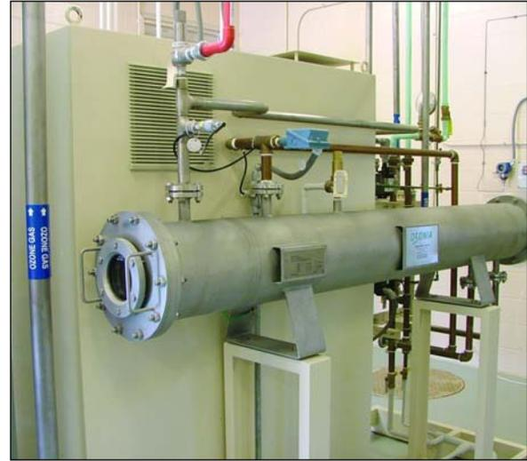
The large capacity "Ozonia" ozone generator is installed in the finished Council Grove water plant, ready to go to work
