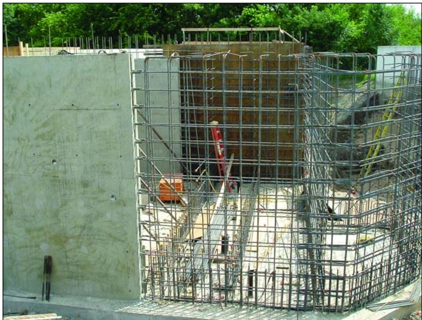
*The steel reinforcement is readied before concrete is poured to form the walls for the ozone generation area of the Council Grove water plant improvement project. CAS Construction, Inc. of Topeka was the general contractor.*
