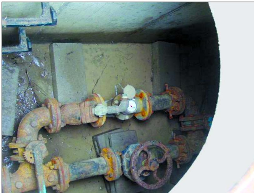
*This master meter and control vault is the point of interconnection for the wholesale purchase of water. In this case, the purchasing system is a small city that serves only 140 services; the seller operates a surface water plant and provides service to 1100 taps.*
