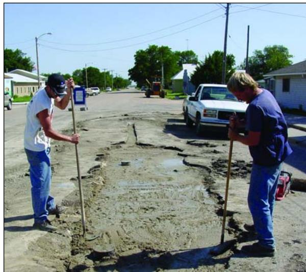
Agra Mayor Scott Bretton, left, and volunteer Melvin Shaffer “puddle the mud” in Main street. Flowable fill, a weak concrete mix, is used on many projects for fast set up and to eliminate settling problems in high traffic areas.
