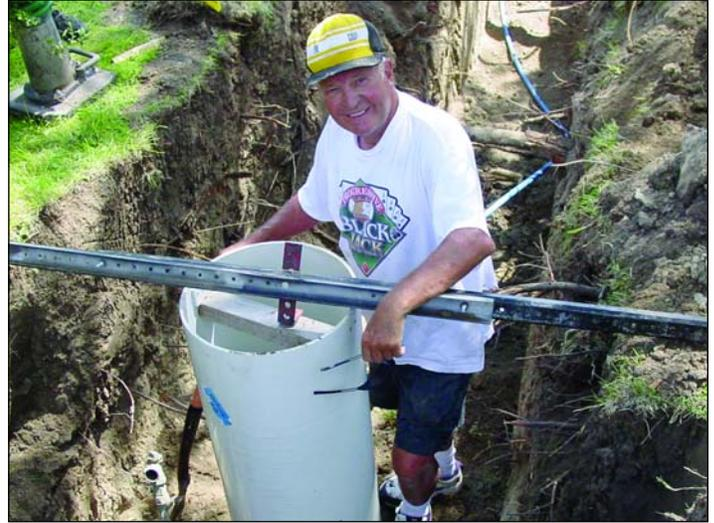
setters/pits. This innovative design allows an operator to maintain the meter and take readings without the help of a flashlight. The 3/4-
