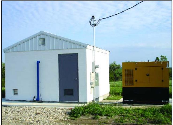
*Brown RWD 1's new pump house north of Fairview replaces a badly deteriorated predecessor that was located at the same location. The new generator at right sits on the original pump house concrete pad.*
