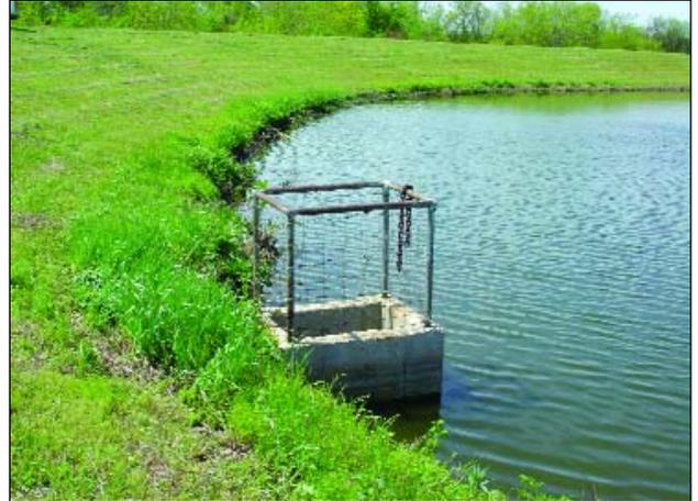
**Left:** Effluent structure photo “before” shown in September 2004 photo. **Right:** Effluent structure “after” photo taken when a new operator had the time to clear the structure of vegetation in order to be able to actually look in to check the system’s effluent.
