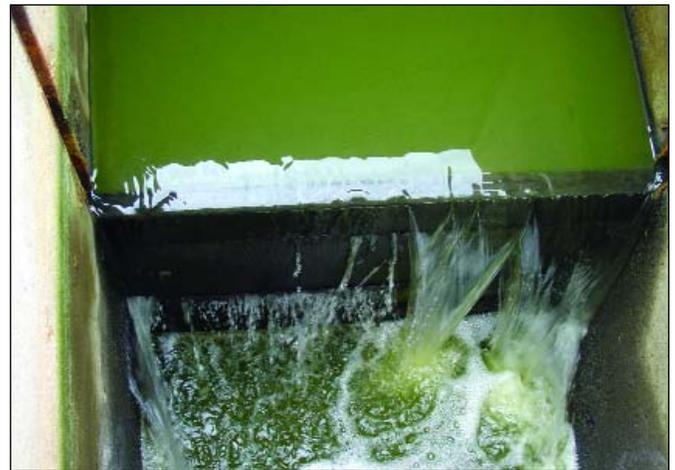
An example of a system's open structure that allows effluent to flow over the top of the weir plates directly from the top of the cell.
