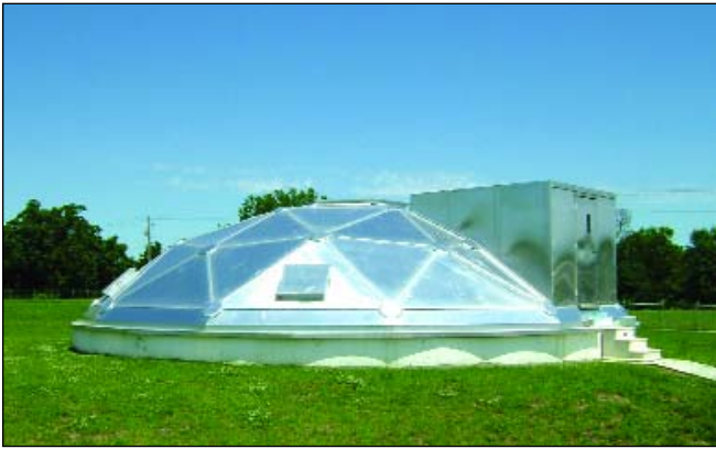
Cover on the north solids contact basin. Note entrance on right and square covers to access/ventilation openings in lower portion of cover
