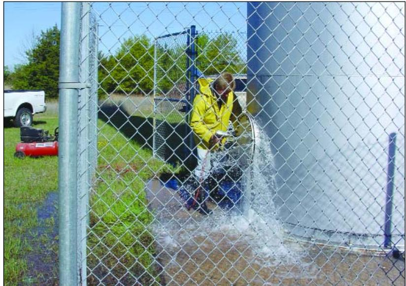
*Steele removes manway cover on the Camp Kanza standpipe in preparation for cleaning which is part of the yearly start-up procedure.*
