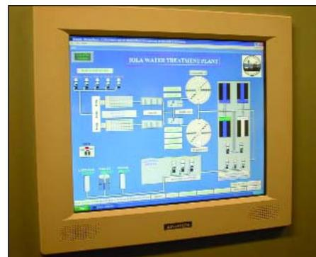
present 1930s era plant, with the addition of ozone and polymers. A new SCADA system has been added. The automated controls should reduce the staffing requirement to have personnel operating the plant eight to 12 hours per day.
