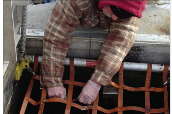
*Jack Fine, City of Winchester, uses latex style gloves to protect against wastewater while working on lift station floats. These gloves can be purchased at local drug store. The safety net is to ensure no one falling into the station.*
