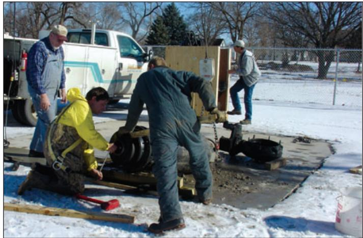
*A crew from Agland Electric, Atkinson, Neb., uses safety harness, rain coat and chest waders while removing and replacing the impeller on lift station pumps at the City of Marysville. Lift stations are confined spaces and proper safety procedures need to be practiced when working on them.*
