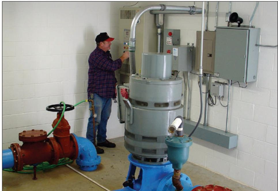
Inside the pump house for Well #3, Larned Water Superintendent Robert Barker adjusts variable frequency drive controllers. There's ample space in this building – a welcome change to many well houses. The drive unit is a 100 hp motor.
